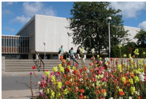
Duncan McArthur Hall, home of the Faculty of Education at Queen's University. (Photo Angela Solar)
